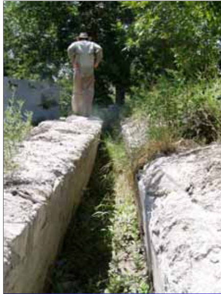
Feeder canal and its 2 nd floor entry to the mill, now at least 10-12 m above the adjacent streambed
